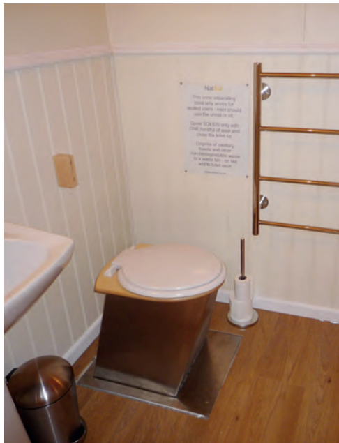
ABOVE Compact, waterless toilets need emptying more often but easily fit into a small cabin or, as here, a shepherd's hut used for glamping holidays at Penn Farm, Devon
